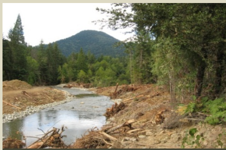
Post-Project: Downstream view immediately after channel construction
