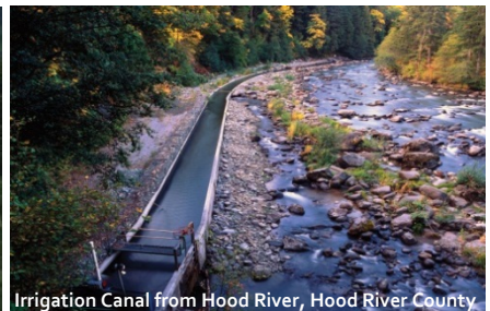
Irrigation Canal from Hood River, Hood River County
