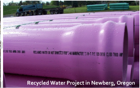
Recycled Water Project in Newberg, Oregon
