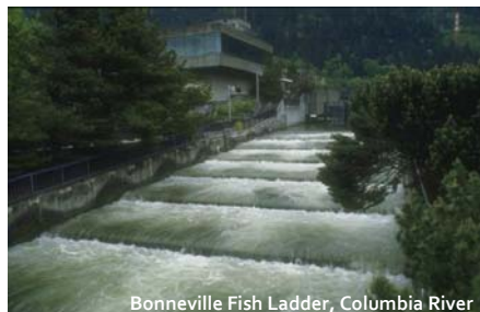
Bonneville Fish Ladder, Columbia River
